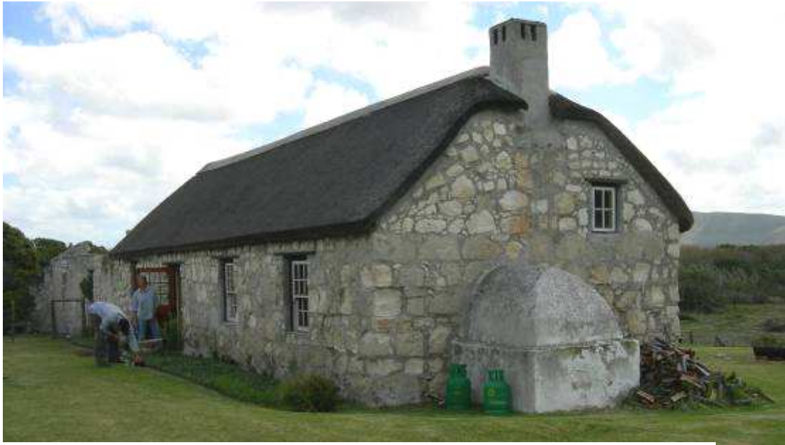
Figure 12 (above) Vernacular cottage at Groot Hagelkraal farm complex. This is a typical Cape “langhuis” built from south coast limestone. The end portion is in a ruined state.
