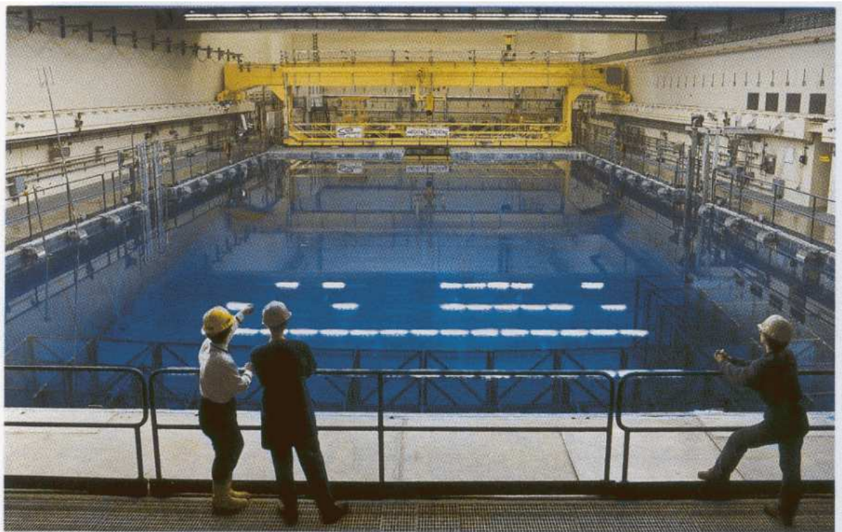
Figure 5.9: An example of a wet storage facility for spent nuclear fuel.
