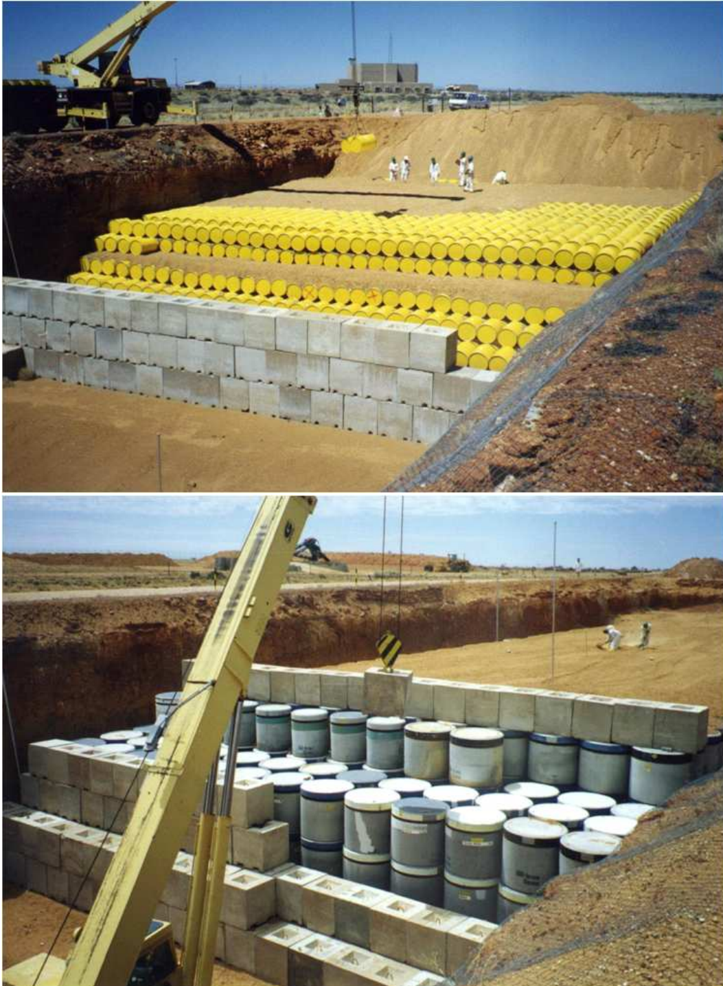
Figure 5.7: Examples of the near surface trenches used for the disposal of LLW (top) and ILW (bottom) at Vaalputs.
