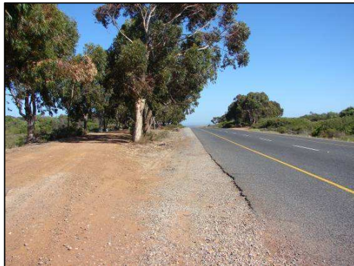
Figure 8.16: North View of a possible traffic lay bye
