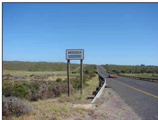
Figure 8.18: Modder River Bridge along the R27
