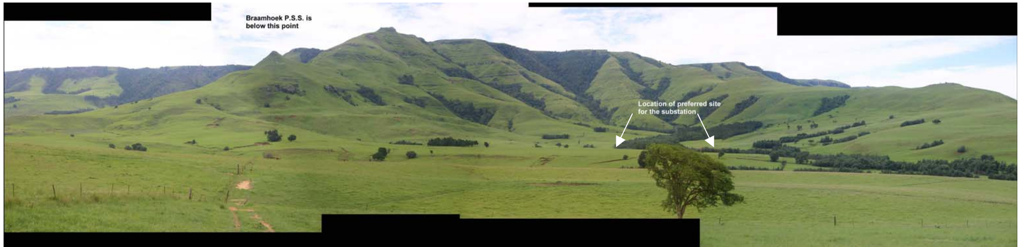
Photo 3: Panorama view of the Braamhoek P.S.S. site location and preferred location of the substation site. (view north)
