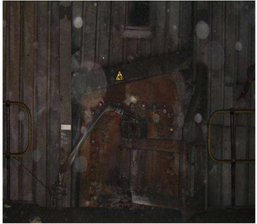
Figure 1 Boiler (lower portion) with the brine injection nozzle
