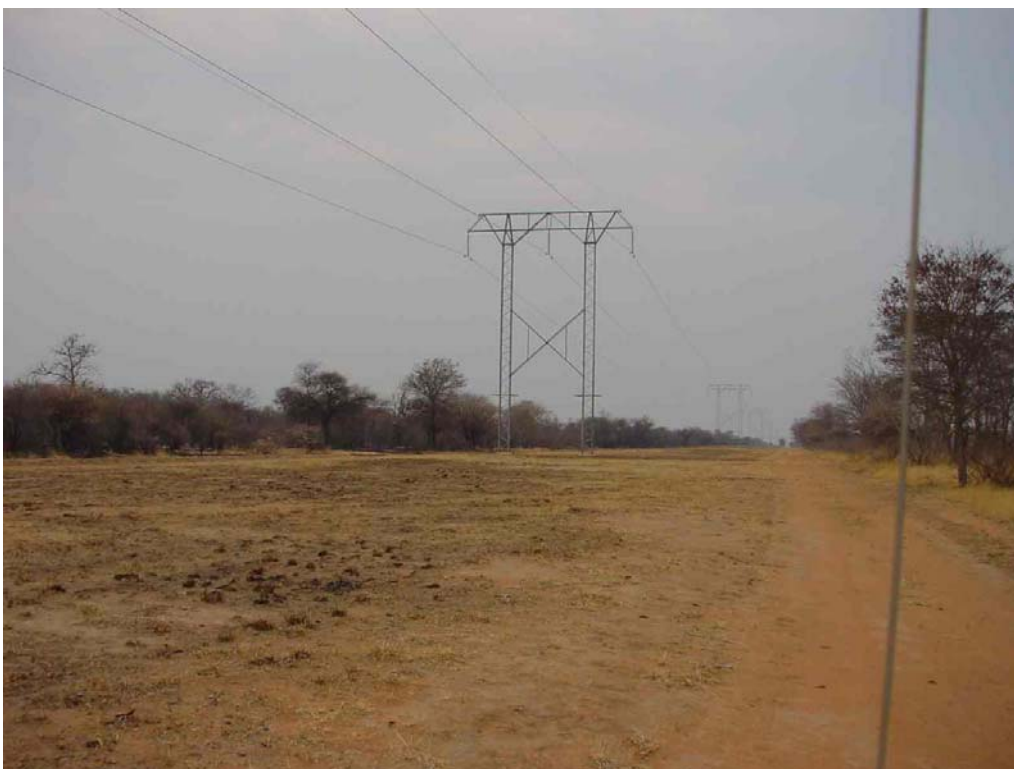
Figure 7. Example of a power line servitude used as a fire break at Thaba Tholo near Thabazimbi.
