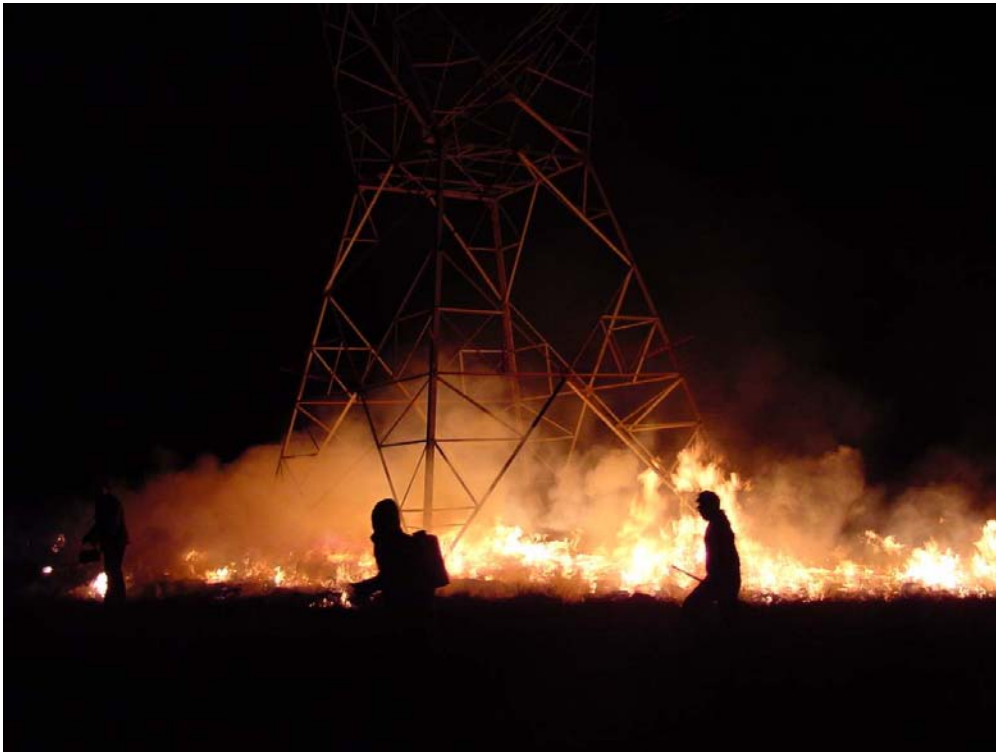
Figure 3 Prescribed burns at night with a low F.D.I. reduces the risk of runaway fires as well as the occurrence of flashovers.
