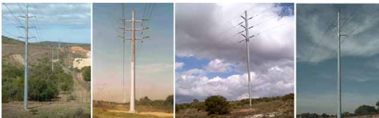
Figure 5.10: Examples of the proposed 132 kV monopole double circuit power line tower type.
