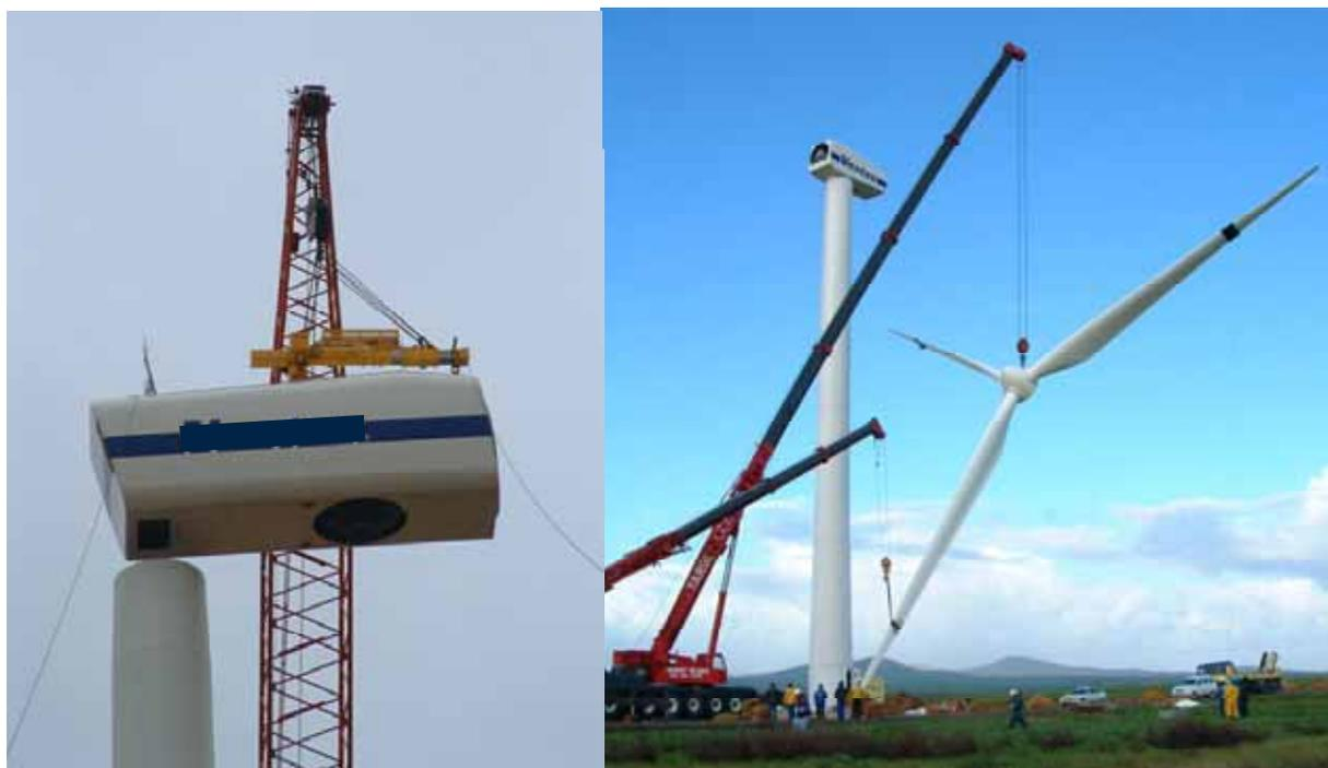
**Figure 7.7:** Photograph illustrating the assembly of a turbine (nacelle and blades) utilising a large lifting crane (photographs courtesy of Eskom from construction at the Klipheuwel demonstration facility)
