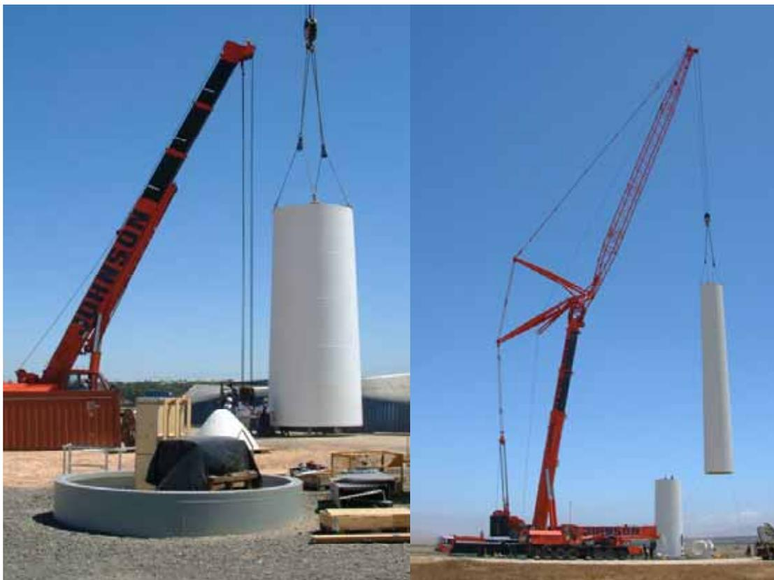
**Figure 7.6:** Photograph illustrating the assembly of a turbine tower utilising a large lifting crane (photographs courtesy of Eskom taken during the construction of the Klipheuwel demonstration facility)
