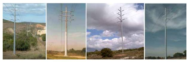
Figure 5.10: Examples of the proposed 132 kV monopole double circuit power line tower type.
