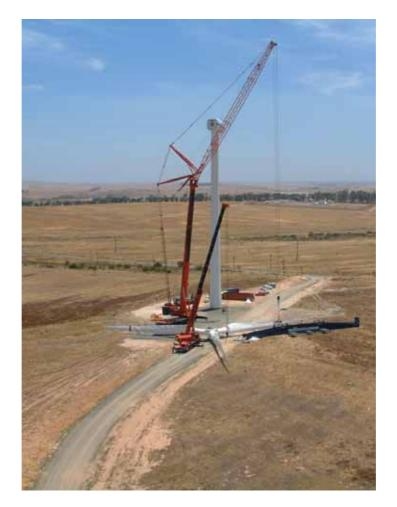
Figure 5.4: Photograph illustrating the laydown areas required during the erection of one of the turbines at the Klipheuwel demonstration facility (photo courtesy of Eskom)
