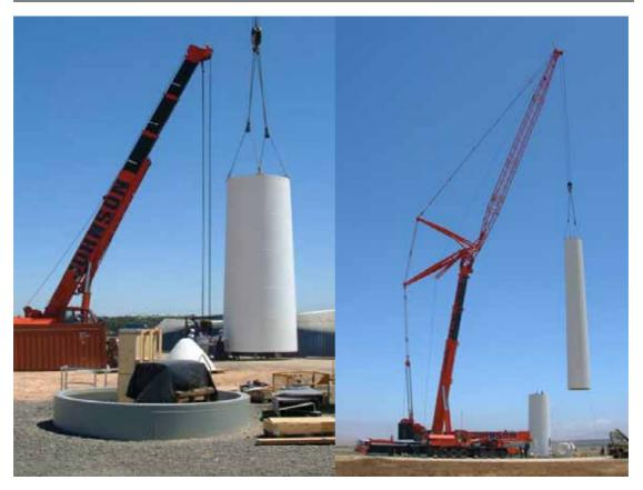
**Figure 5.7:** Photograph illustrating the assembly of a turbine tower utilising a large lifting crane (photographs courtesy of Eskom taken during the construction of the Klipheuwel demonstration facility)
