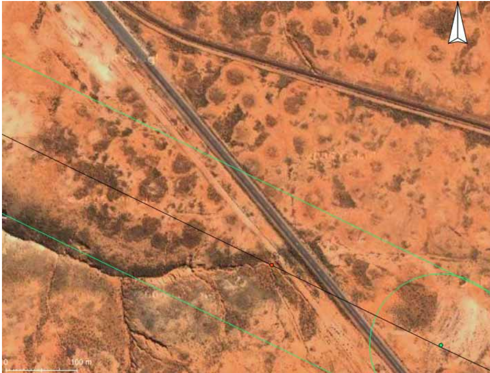
Figure 15. Erosion gully network. Most of the area in close proximity to the drainage line is likely to be highly susceptible to sheet, rill or gully erosion. Towers located in this area could be undercut by the erosion. Runoff from roads could exacerbate erosion in the area.
