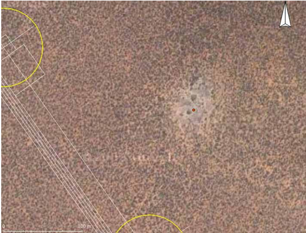
Figure 27. Enigmatic feature within the area occupied by the WEF. The feature may represent a pan. In terms of the current layout it would appear to lie in excess of 50 m of any infrastructure.
