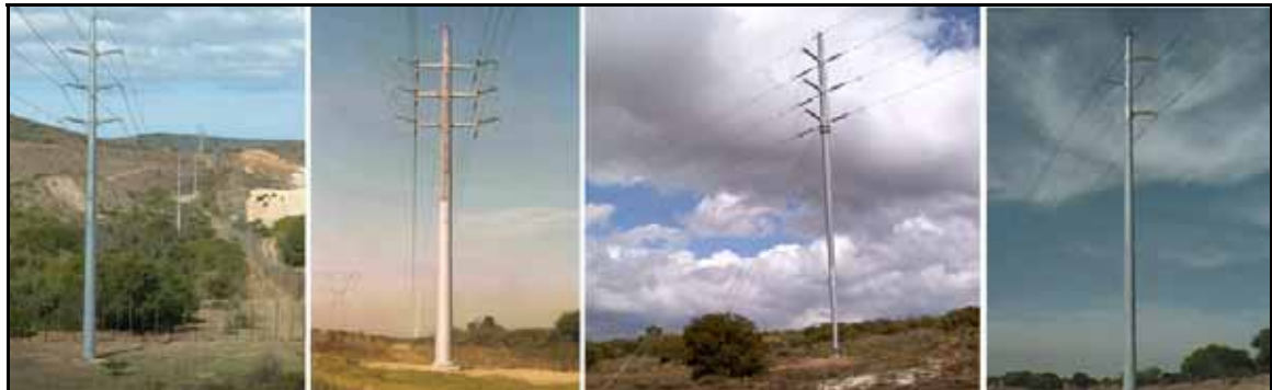
Figure 9: Examples of monopole transmission line towers
