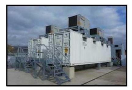
Figure 2-2: An example of a lithium-ion container installation
