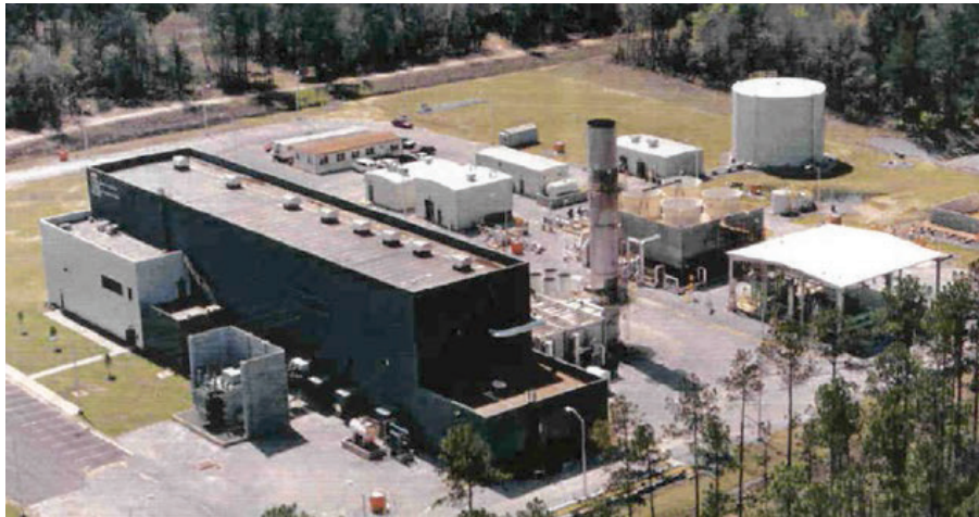
Power South McIntosh AL, CAES plant has been online since 1991
