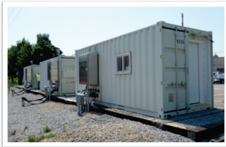
1-MW electrochemical capacitor regenerative braking system provides 20-second charge and discharge cycles [0365]
