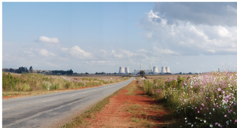
View 13: Kendal Power Station
