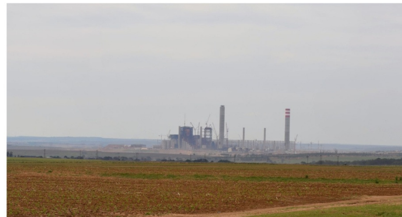
View 14: Kusile Power Station, currently under construction
