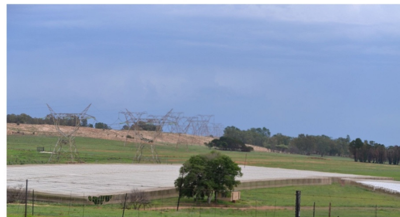
View 16: power lines
