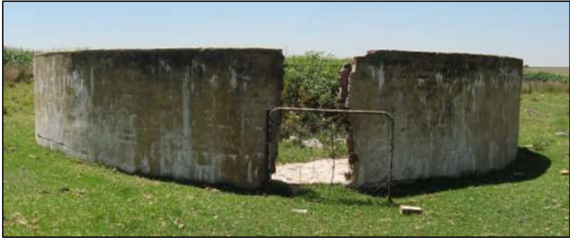
Figure 17 – Site A2, brick and cement dam
