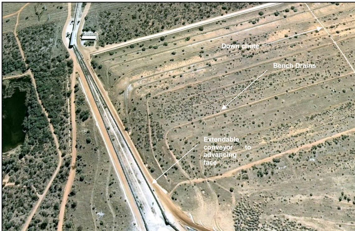
Figure 13: Plan view of rehabilitated ash stack at Matimba Power Station Ash Facility
