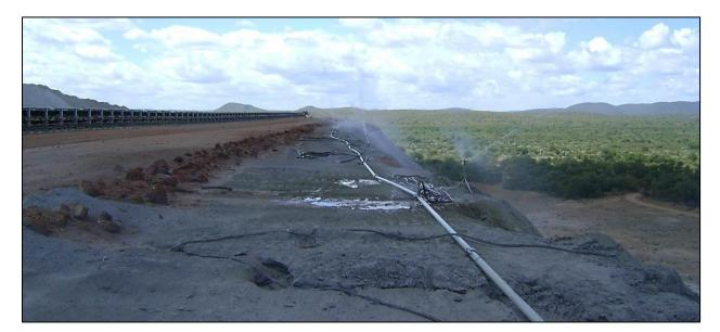
Figure 8-11: Dust suppression system at Matimba Power Station
