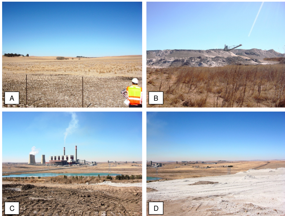
Figure 4-6: Photographs taken during the screening/scoping survey: facing south towards the pan and channelled valley bottom system (A); facing north at the existing ash disposal facility on the 35 year ashing line (B); facing east toward a dam and the Majuba Power Station (C); and facing southeast at the tributary of the Witbankspruit.
