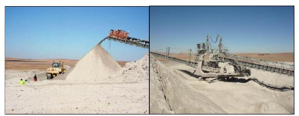
Figure 7.1: Stacker being used to dispose of ash at the Majuba Power Station
