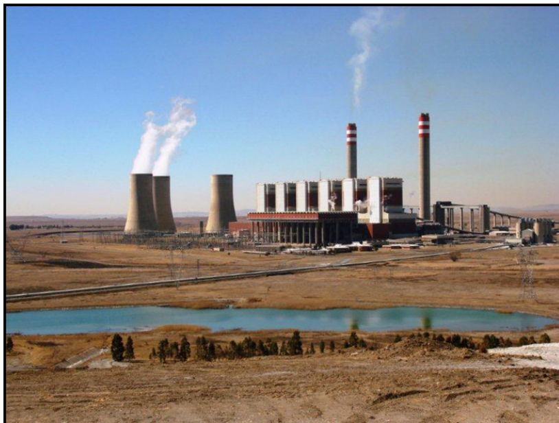
Figure 2: Majuba Power Station forms the centre point of the study area.
