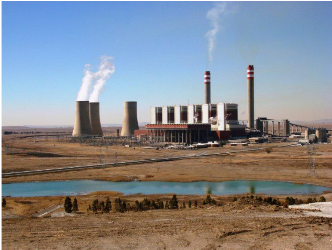
Figure 10.3: Majuba Power Station forms the centre point of the study area
