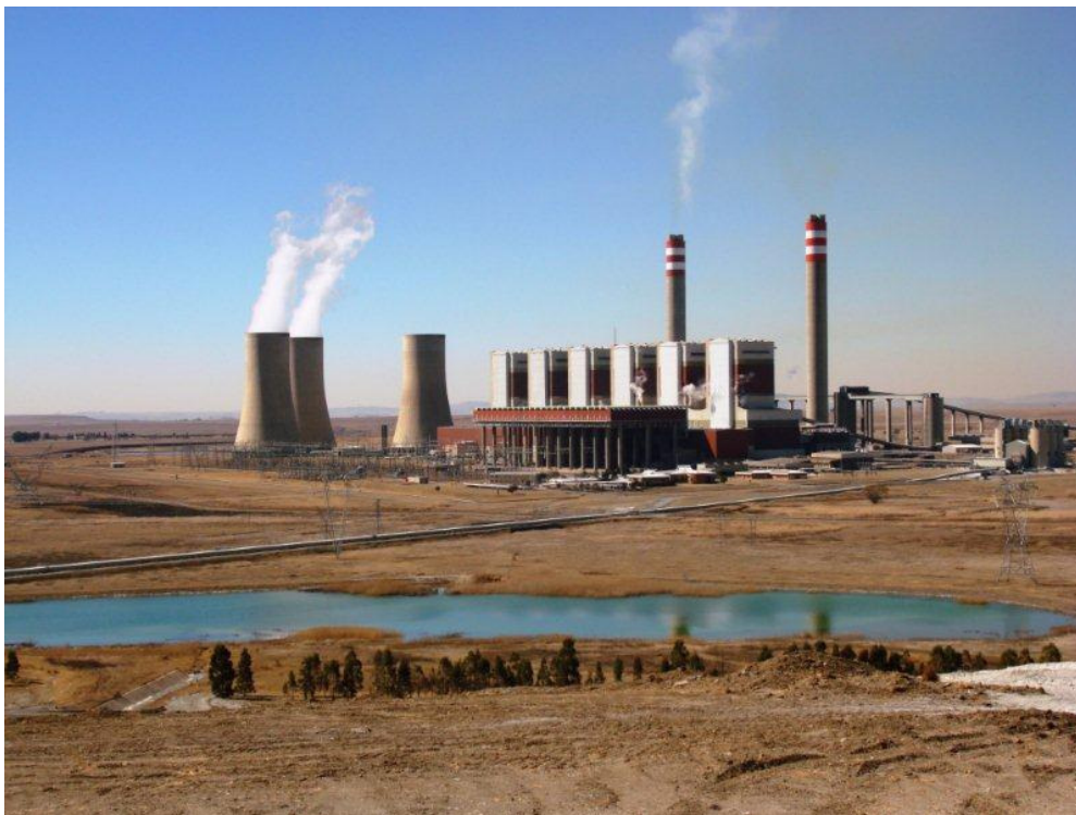
Figure 4.2: Majuba Power Station forms the centre point of the study area
