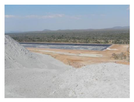
Photo 15.1: Site Alternative 1 - Lined PCD under construction taken from the existing Matimba Ash disposal facility
