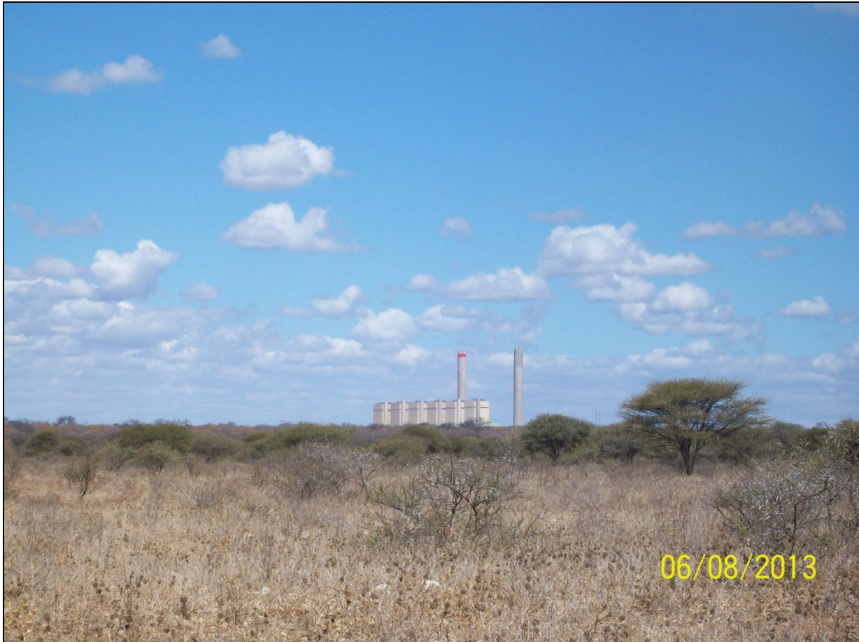
Figure 36: Matimba Power Station, as seen from site alternative two
