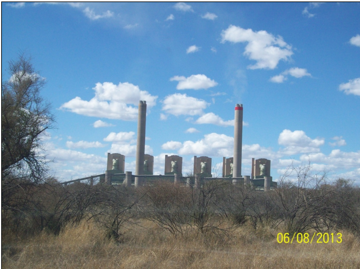
Figure 25: View of Matimba Power Station from Road D6175
