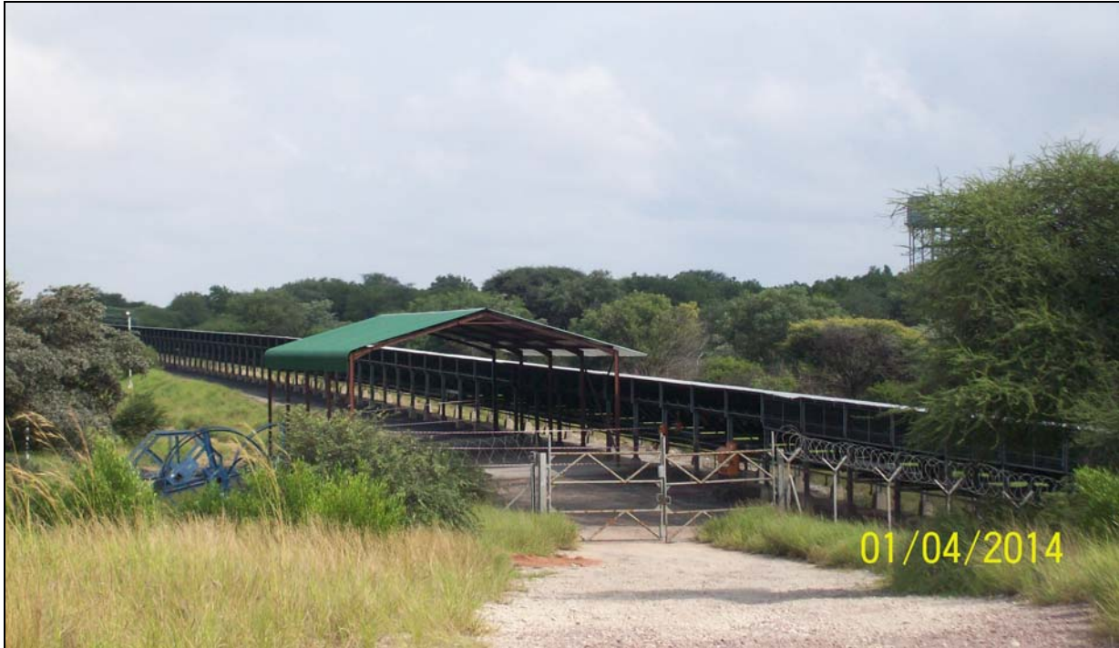
Figure 33: Example of a conveyor belt carrying coal from Grootegeluk Mine to Matimba Power Station
