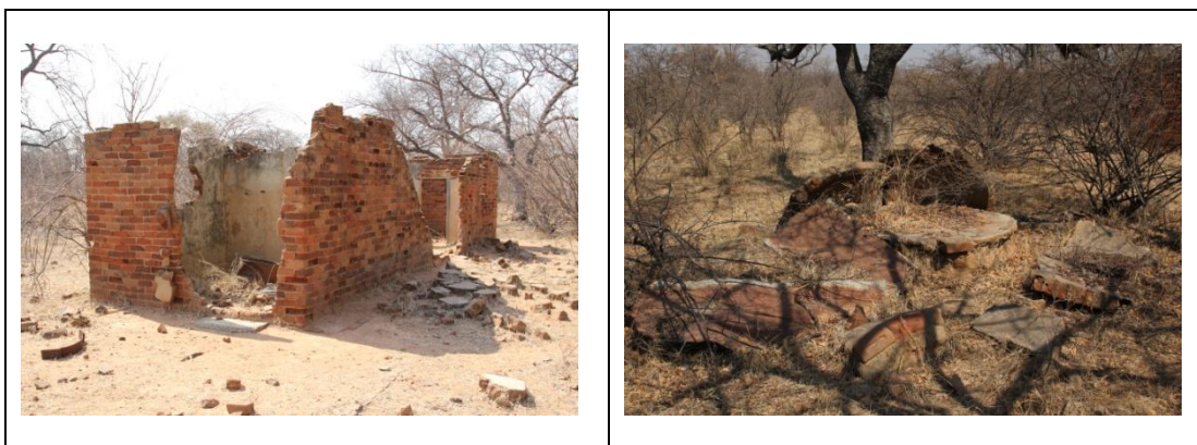
Figure 14: The remains of the old house structure.
