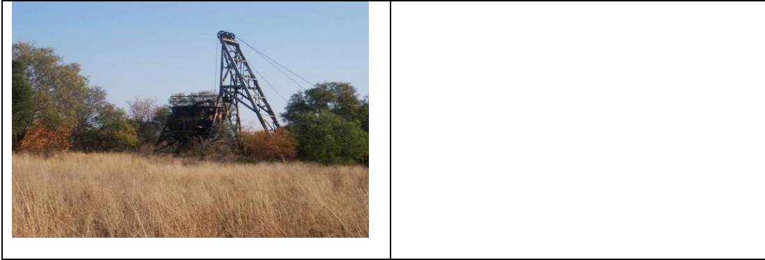
Figure 12: Head-gear of the first mine shaft that was sunk in the region.
