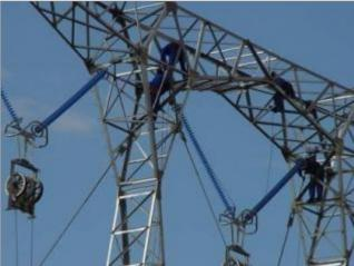
Figure 29: Stringing with pilot tractor (top) and pulleys (bottom)
