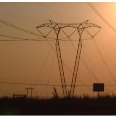
Figure 15: Guyed suspension tower
