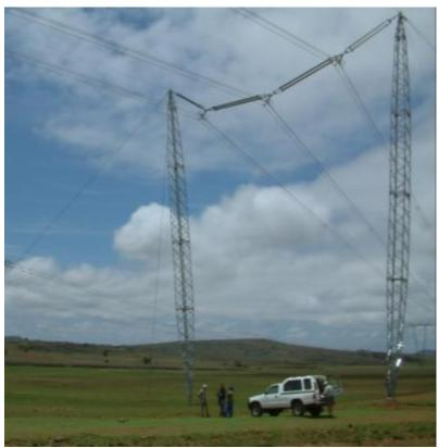
Figure 13: Cross-rope suspension tower
