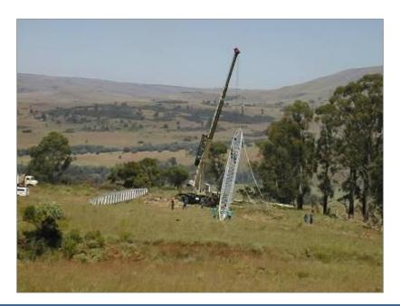
Figure 27: Erection of towers
