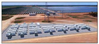
Figure 5: Example of a BESS
