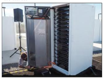
Figure 6: Solid state battery module
