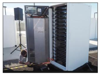
Figure 6: Solid state battery module
