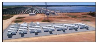
Figure 5: Example of a BESS
