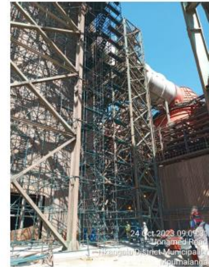
Figure 9: Lobster Unit 2 – Access Scaffolding
