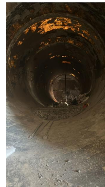
Figure 15: Unit 1 – Horizontal Duct Cleaning
