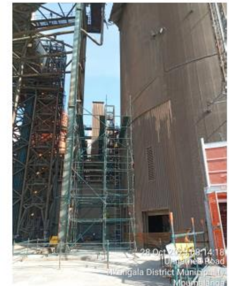
Figure 10: Lobster Unit 1 – Access Scaffolding
