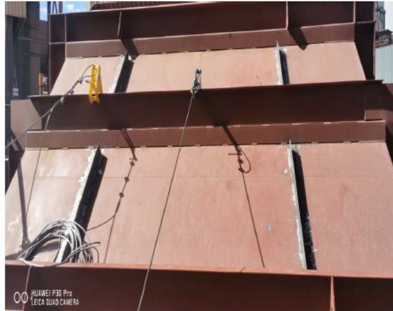
Figure 23: East Side – Roof Strengthening Completed
