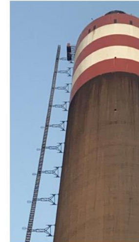
Figure 9: Alimak – Landing platform and gates installed
