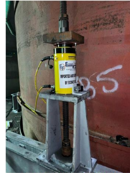
Figure 5: 180m platform – Jacks complete with Stroke sensor connected to Power Pumps
