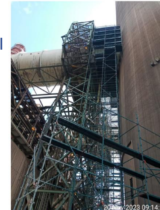
Figure 4: Unit 2 – Access Scaffold Erection
