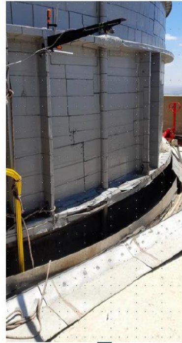
Figure 6: 211m Roof – Draw-wire to Measure Flue Displacement
