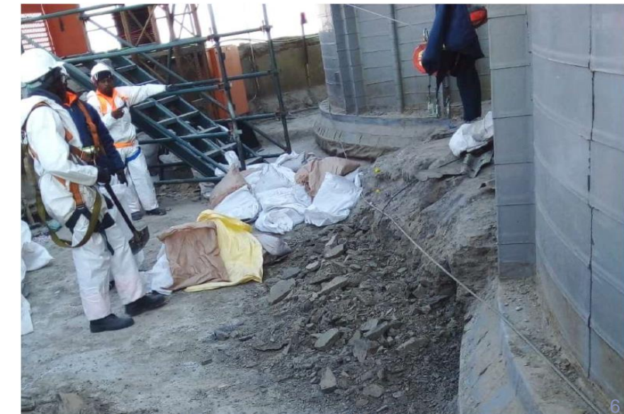
Figure 6: 211m Roof – Removal of Slurry
