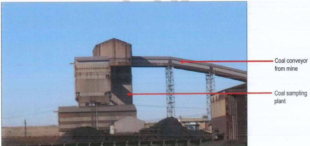
Figure 3: Coal sampling plant with coal conveyor
