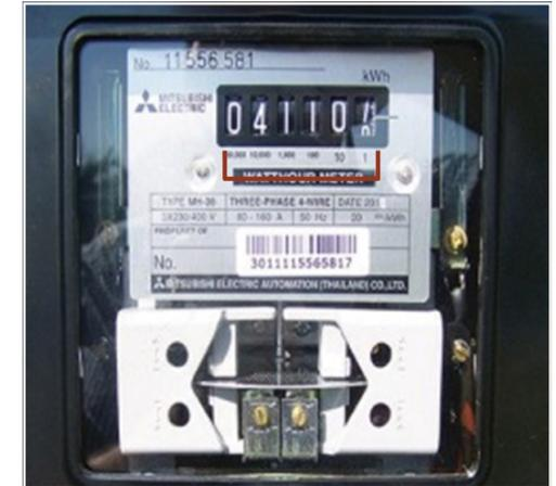
Figure 4: Mitsubishi kWh meter with 6 numbers. This reading would be 041107
