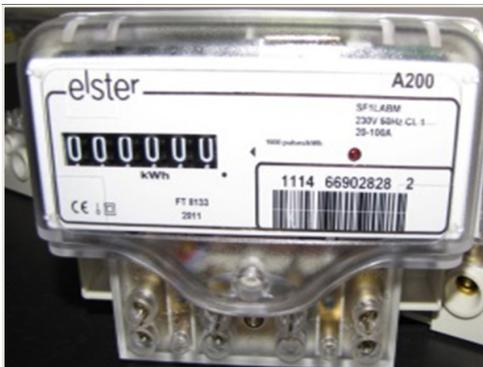
Figure 5: Elster kWh meter with 6 numbers. All 6 of the numbers must be read including any zeros before the comma. This reading would be 000000
