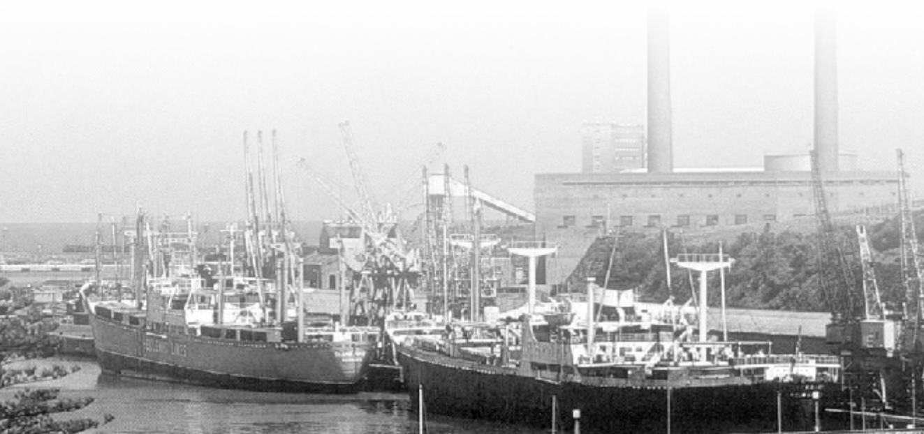
~ West Bank Power Station
