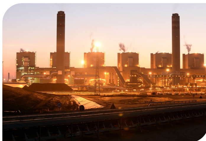
Medupi Power Station
