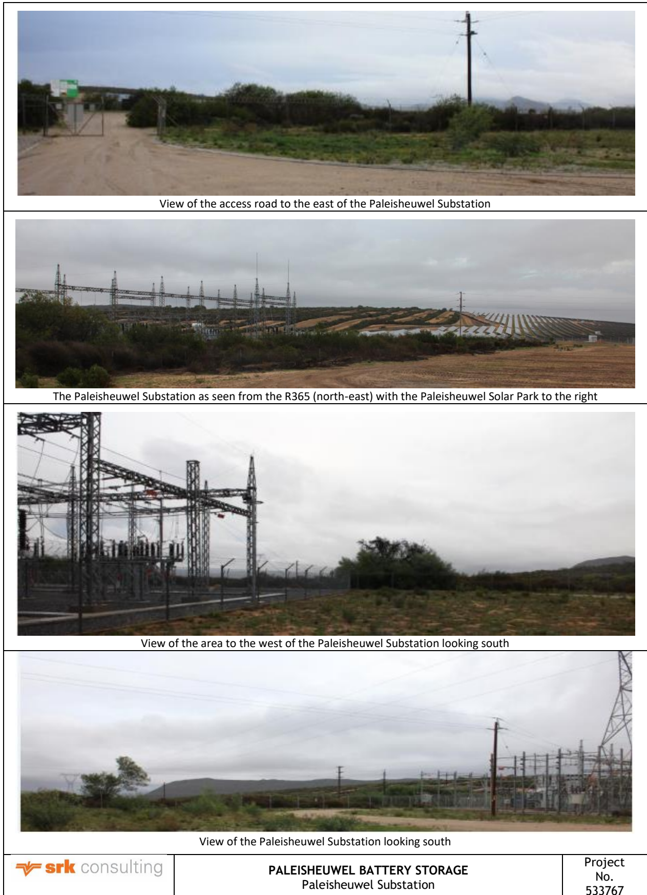
Figure 1-4: The Paleisheuvel Substation as seen from various viewpoints
