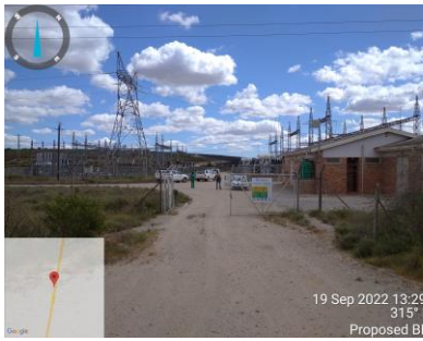
Photo of the entrance to Paleisheuvel Substation
