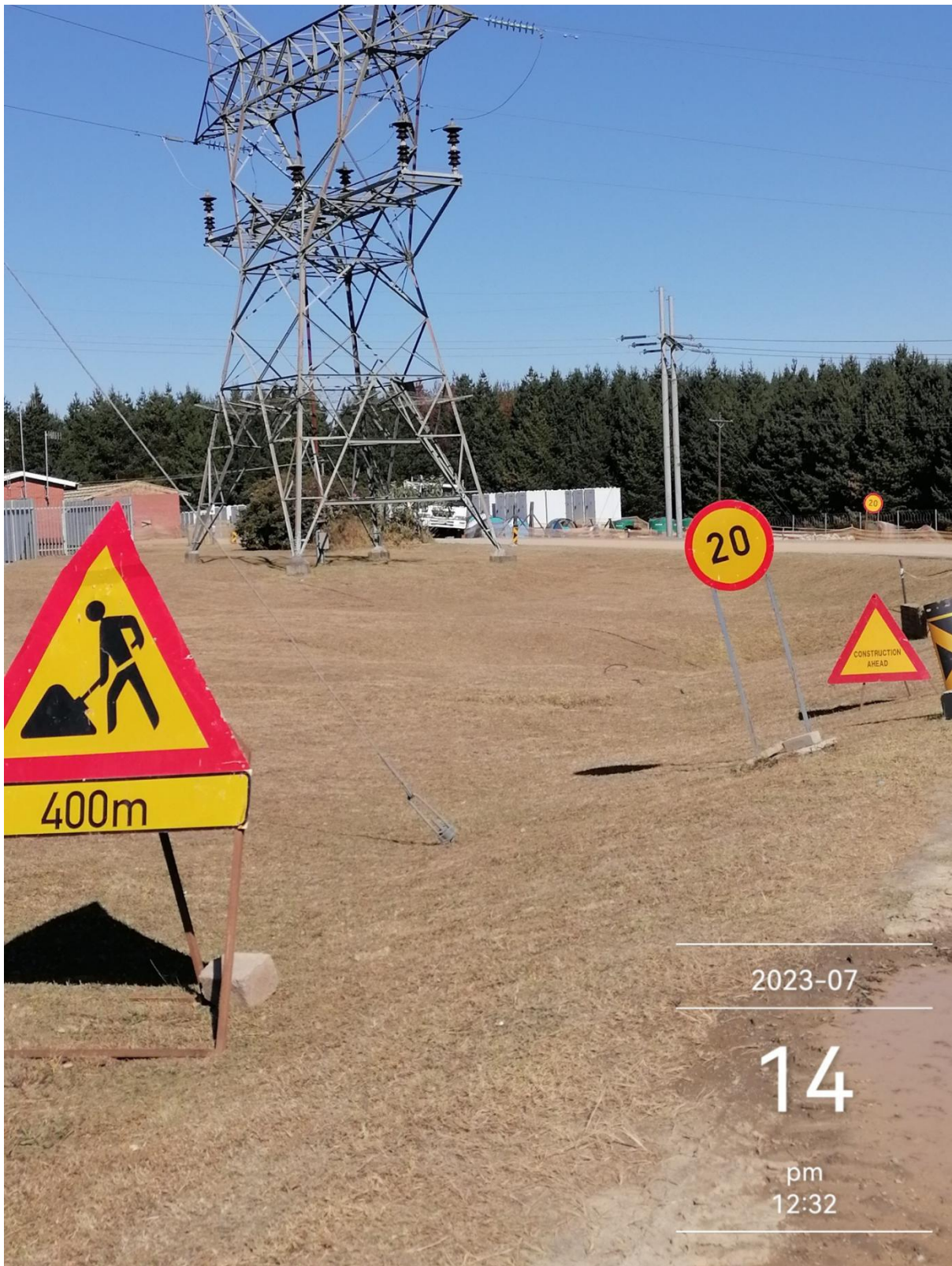
Figure 5: Site Garden and landscape well maintained
