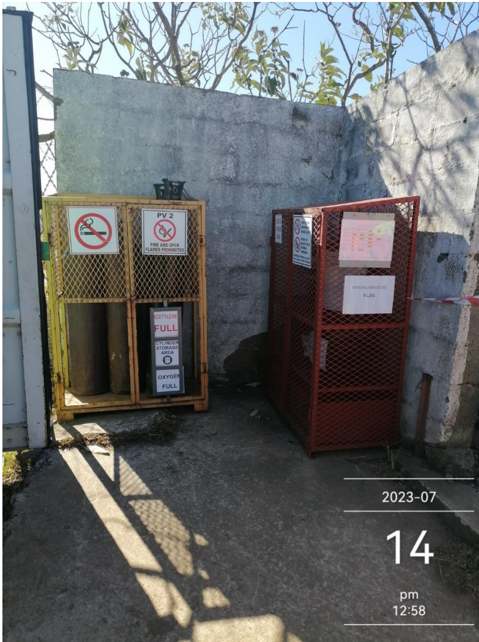
Figure 4: Gas Bottles and other chemicals are safely secured in safe cages
