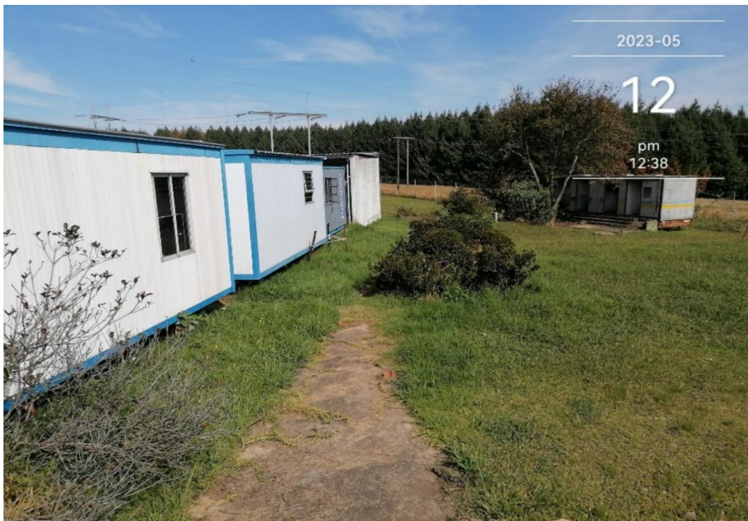
Figure 6: Site Garden not maintained
