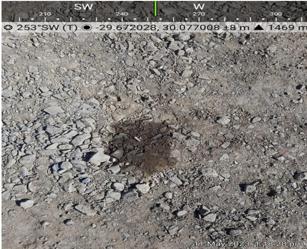
Figure 12: Showing the minor oil spill observed from a TBL on side
