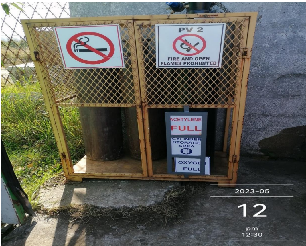
Figure 3: "No open flame" signage and cages well secured
