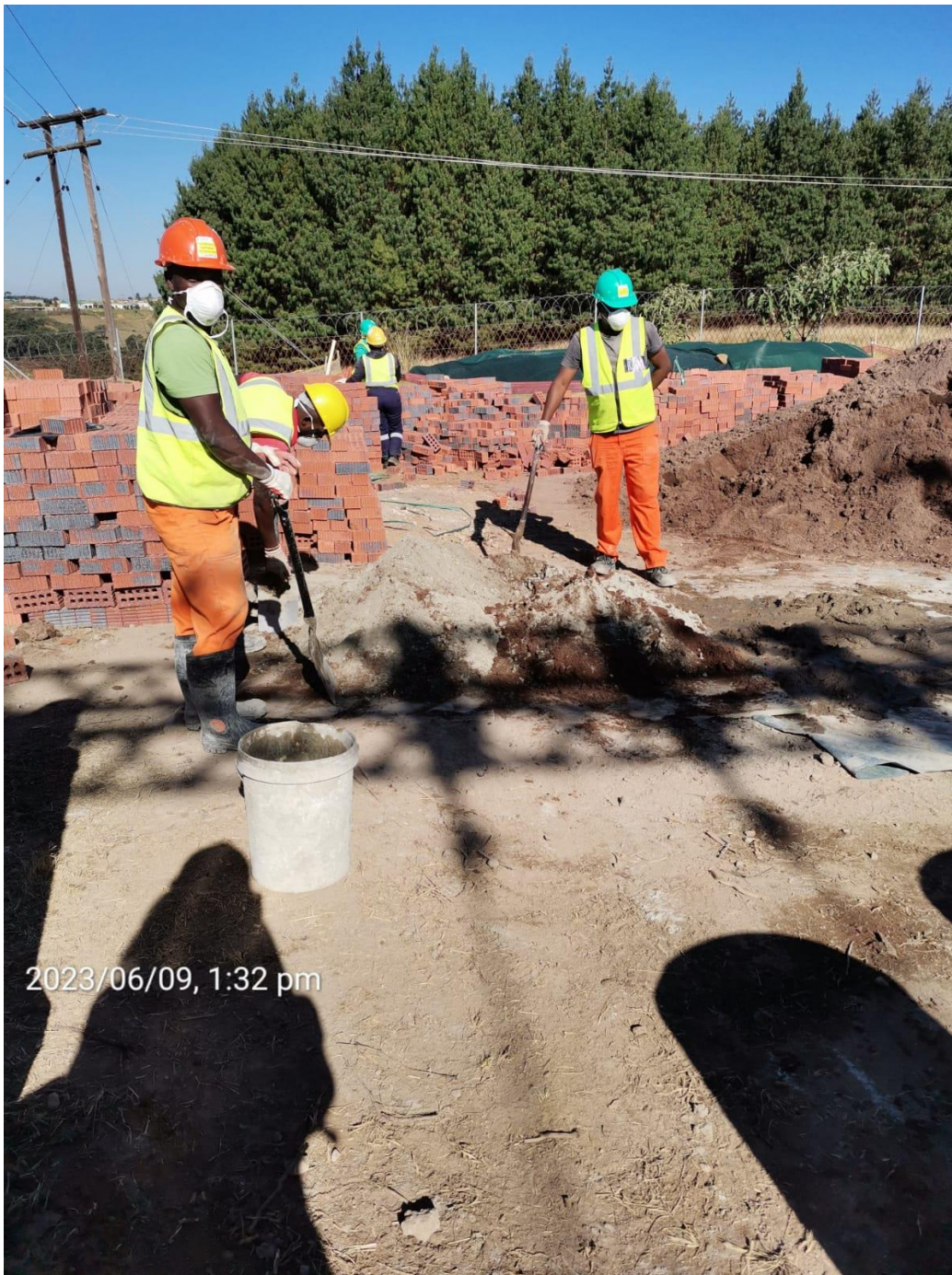
Figure 1: Cement mixed on plastic to prevent soil contamination
