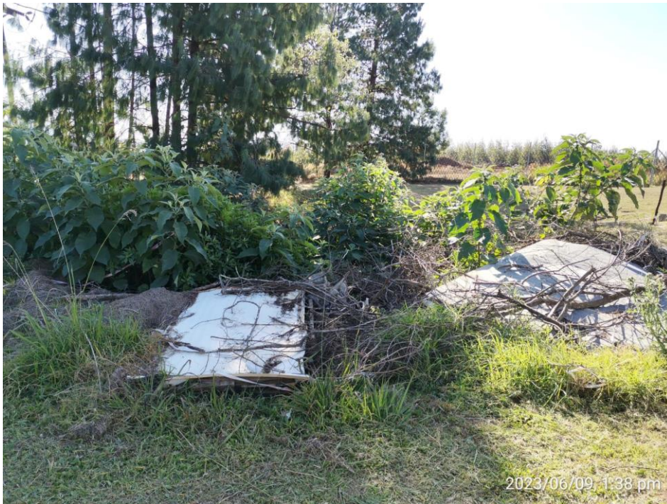
Figure 4: Mixed waste not collected at the back of the site office since start of construction
