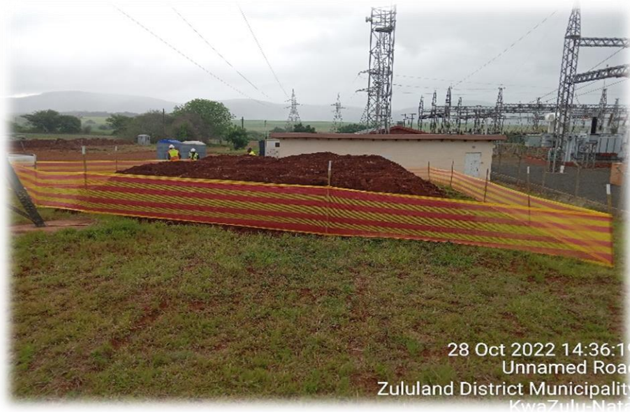
Picture 3.6.1. Shows an area demarcated for top soil stockpiling.
