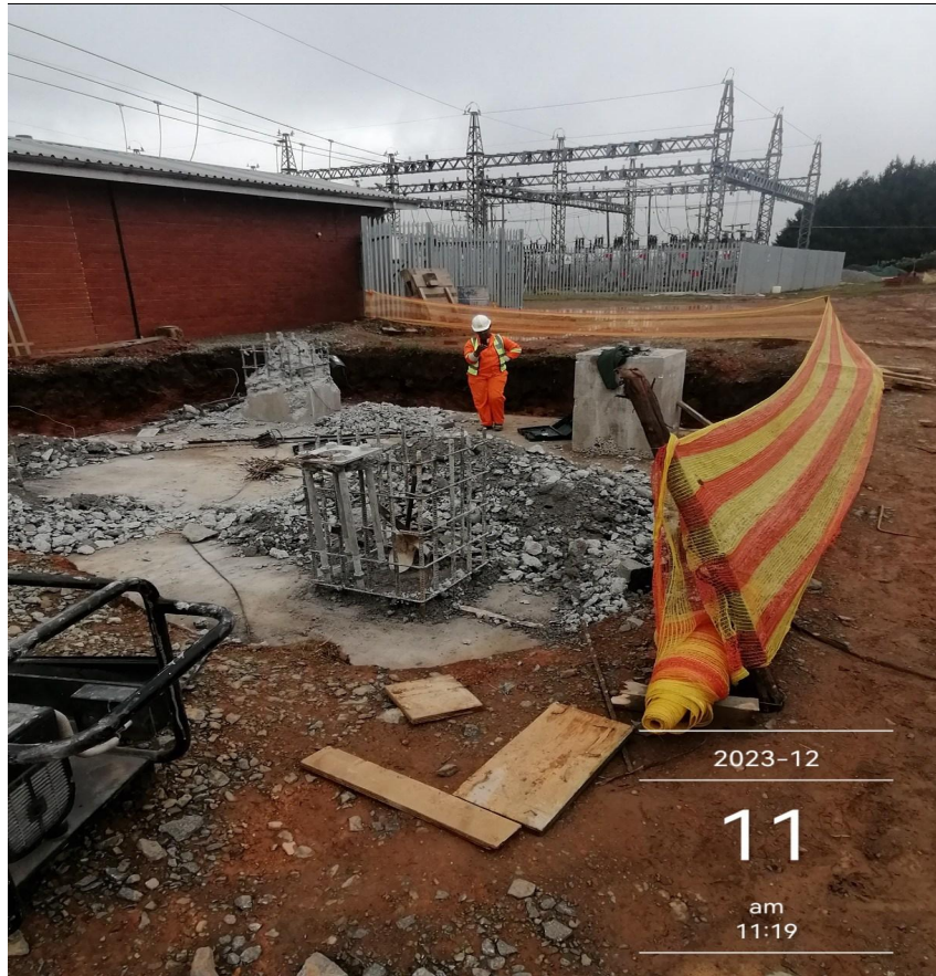
Figure 3: Excavation with appropriate demarcation nets
