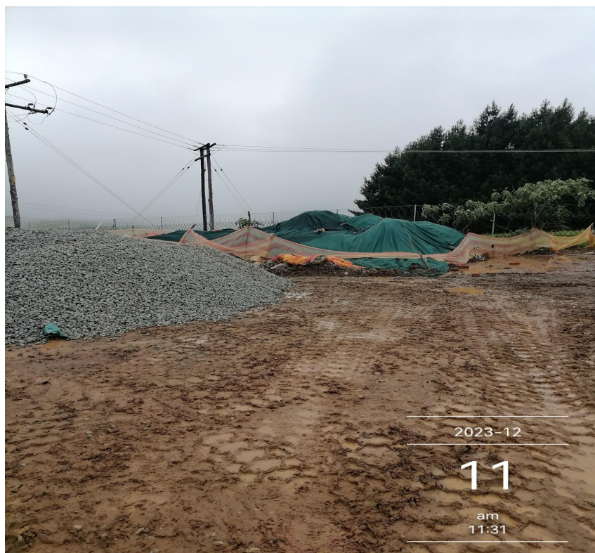
Figure 4: Topsoil separated, heaped and covered as required
