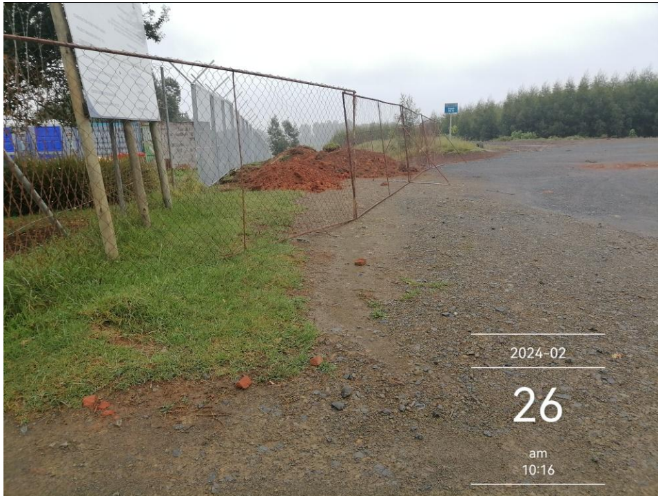
Figure 3: Precinct Fence Installation trenches properly demarcated
