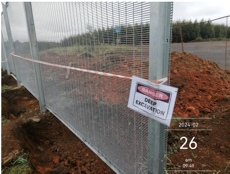
Figure 12: Excavations clearly marked and demarcated
