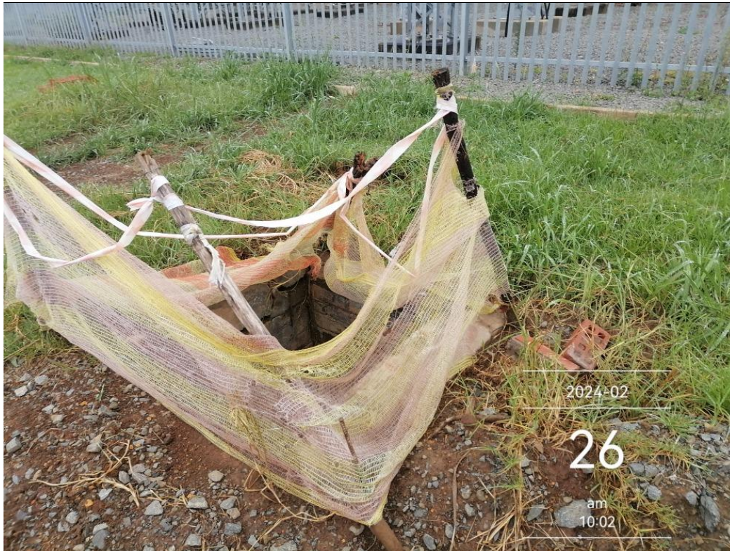
Figure 9: Storm water pit demarcated
