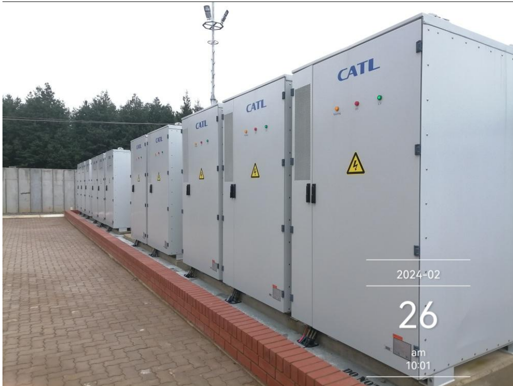
Figure 7: The battery area properly paved and clean
