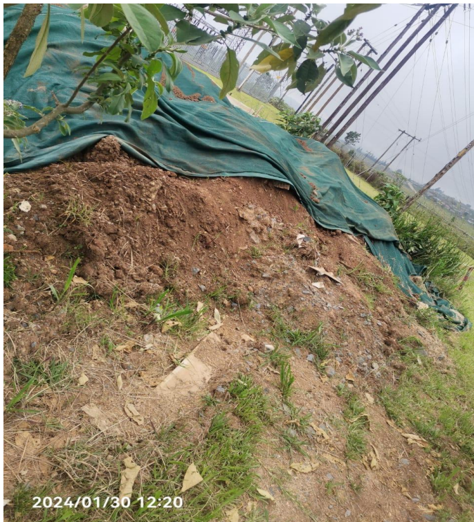
Figure 1: Top Soil not fully covered
