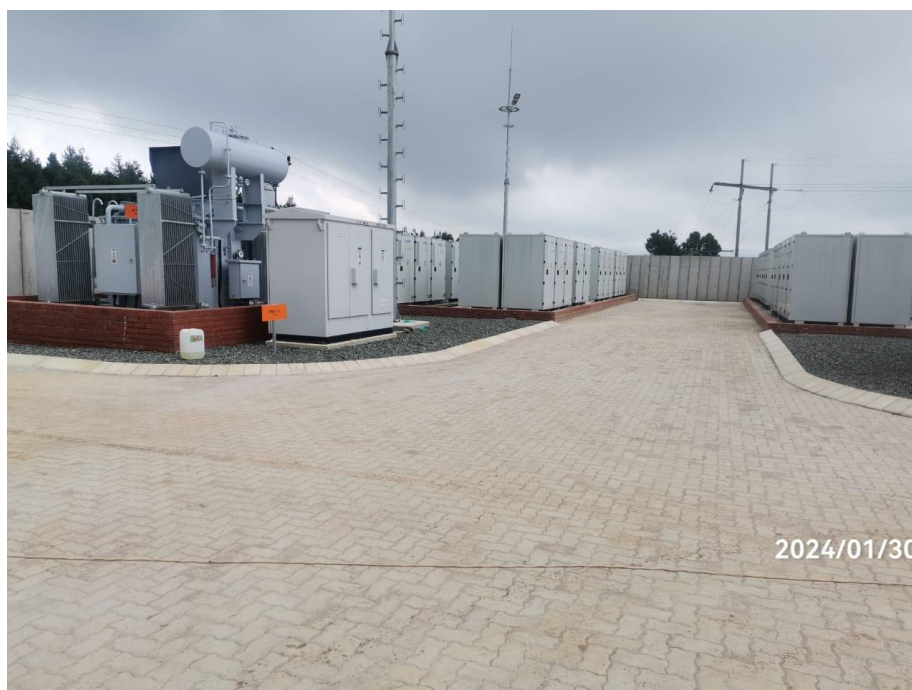
Figure 6: Appropriate paving inside the battery yard
