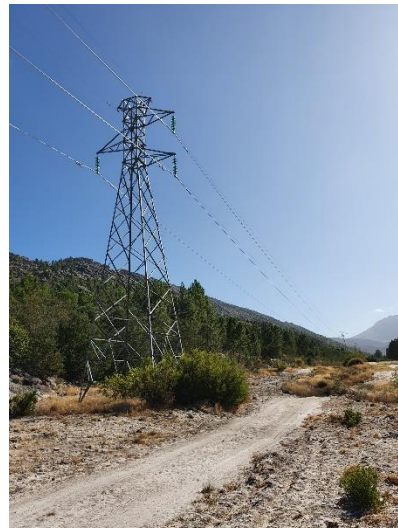
Plate 1d: Disturbed areas and natural vegetation surrounding existing access routes
