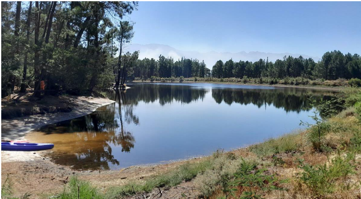
Figure 3: Dam in the PAOI.
