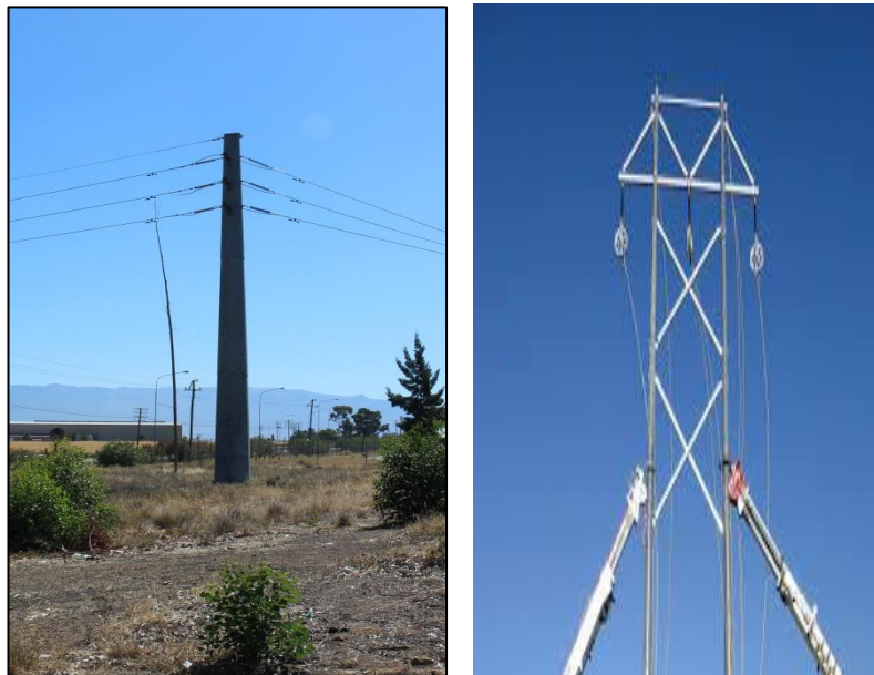
Figure 3-1: Indicative representation of the pylon types considered for the project - steel monopole (left) or braced double steel poles (right)
