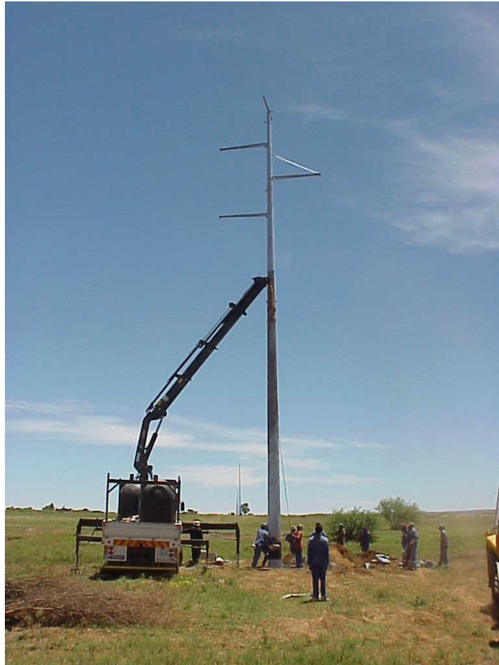
Figure 2: Installing Power Line
