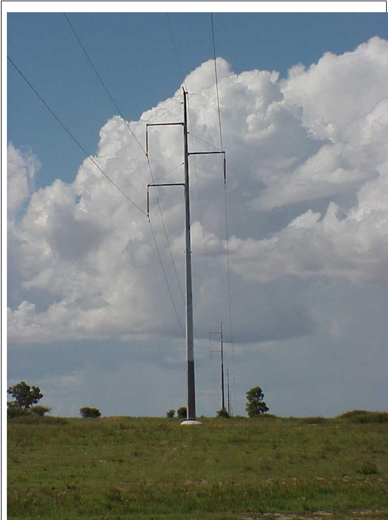
Image of Eskom 132kV bird friendly mono pole structure
