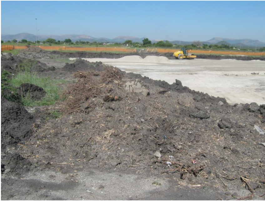
Photo 5: Topsoil being preserved for future rehabilitation purposes.
