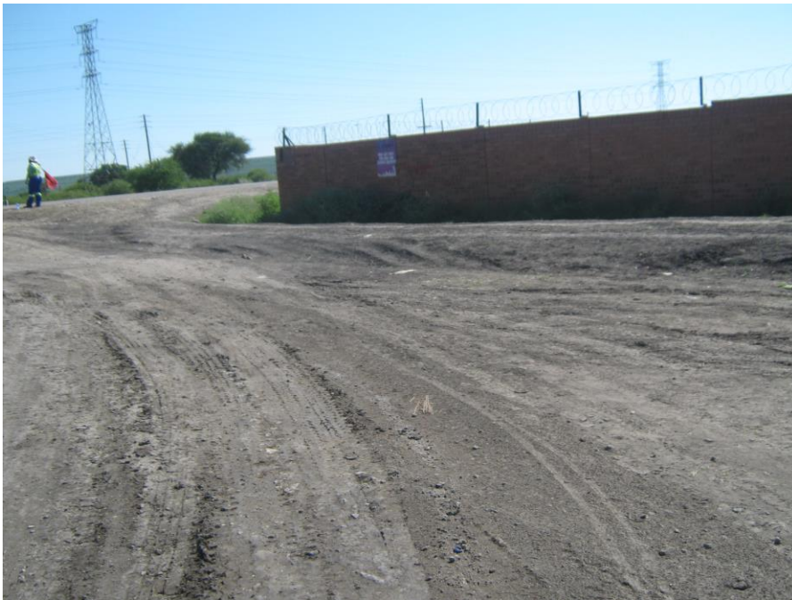
Photo 6: A storm water diversion berm near the site camp entrance.
