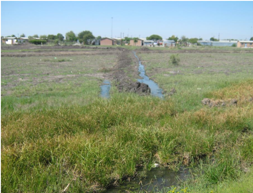
Photo 10: A cut-off trench on the west side of the construction site.
