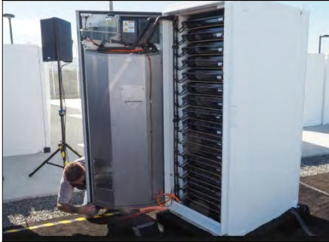
Figure 6: Solid state battery module
