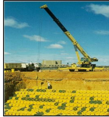
Figure 3-17: Placement of Low Level Waste steel drums at Vaalputs
