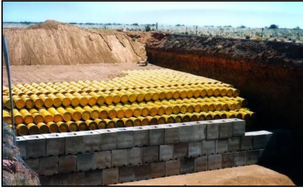
Figure 3-16: Low Level (steel) and Intermediate Level (concrete) radioactive waste drums (respectively above and below) at Vaalputs. The drums are covered with layers of clay.
