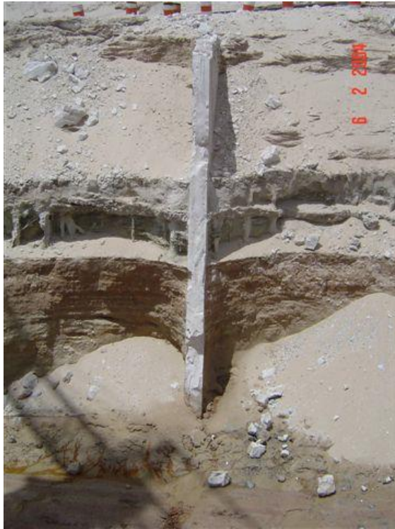
Figure 10-1: Example of cut-off wall used at Coega Harbour
