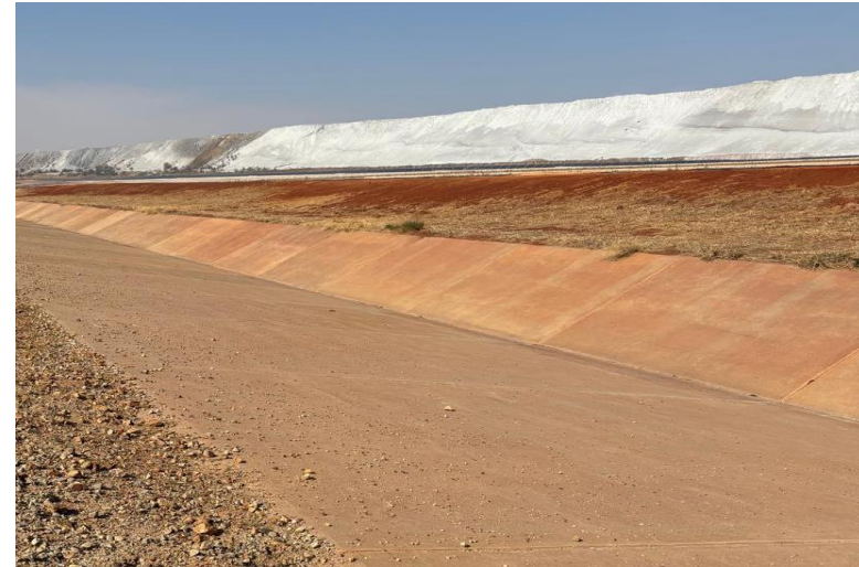
Figure 6 Clean V-Drain
