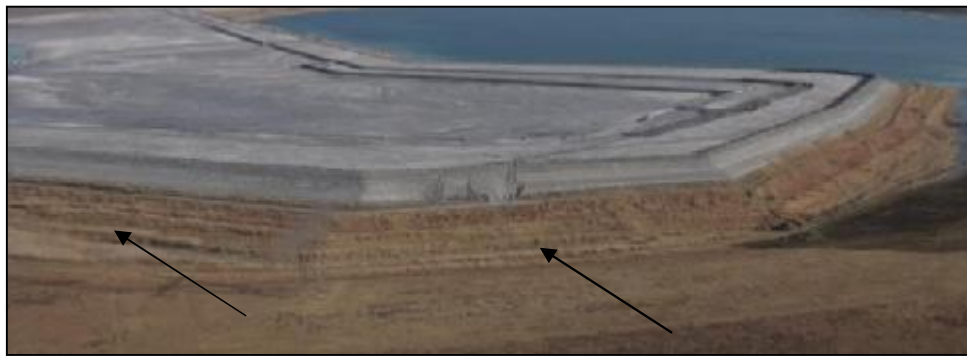
Figure 3-4: Existing ash disposal site with capped and rehabilitated area in the foreground
