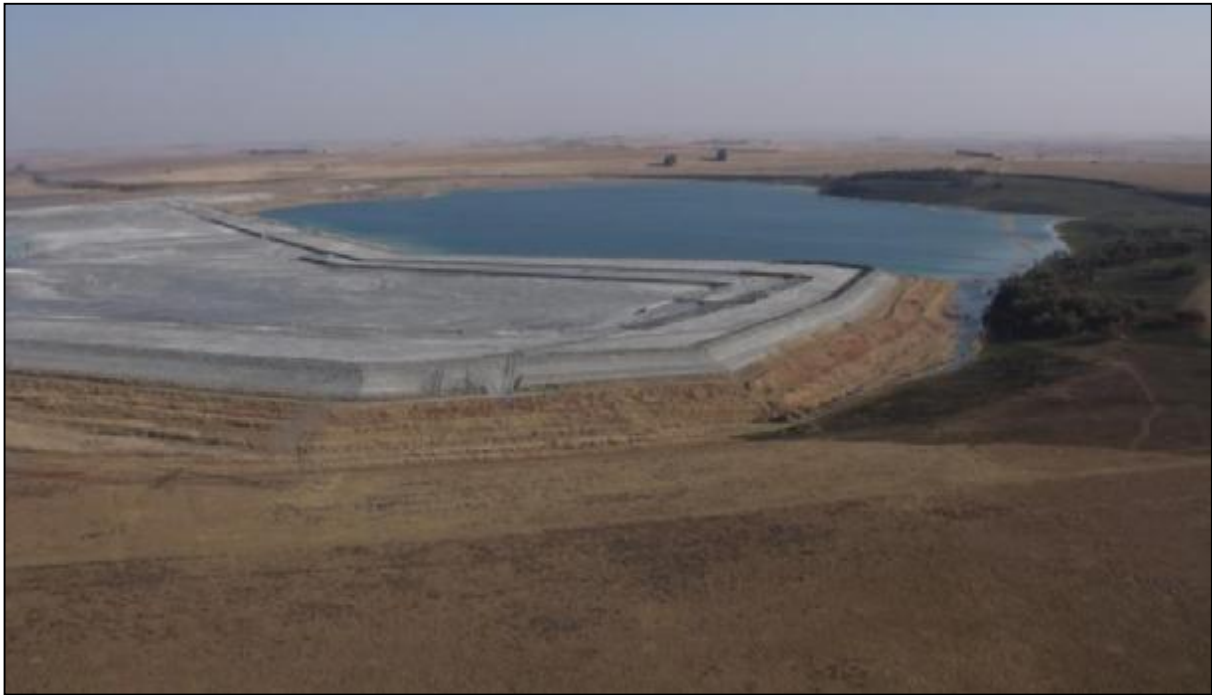
Figure 3-2: View of the sides of the existing ash disposal site.
